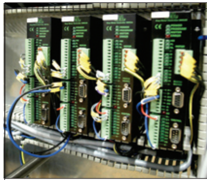
Step Motor Controllers SMC35 in the machine's control panel.
